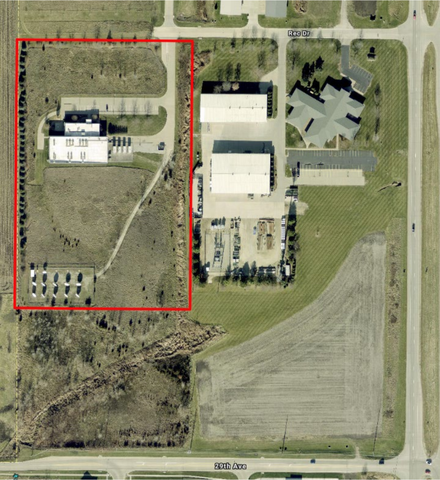
Ark Data Center Campus – Marion, IA
