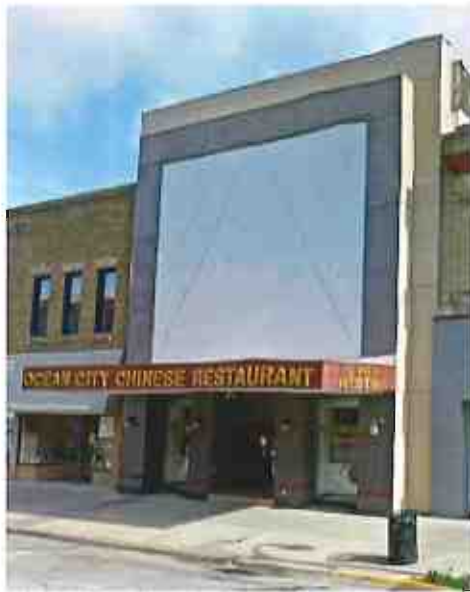
5 West Main Street before renovation
