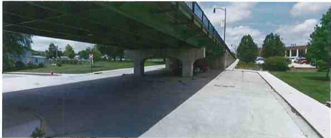
Existing conditions under the Center Street bridge
