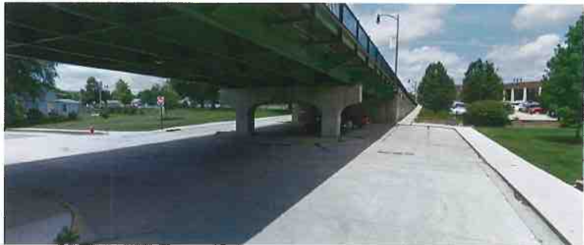
Existing conditions under the Center Street bridge
