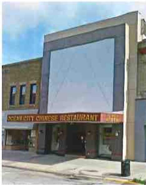
5 West Main Street before renovation
