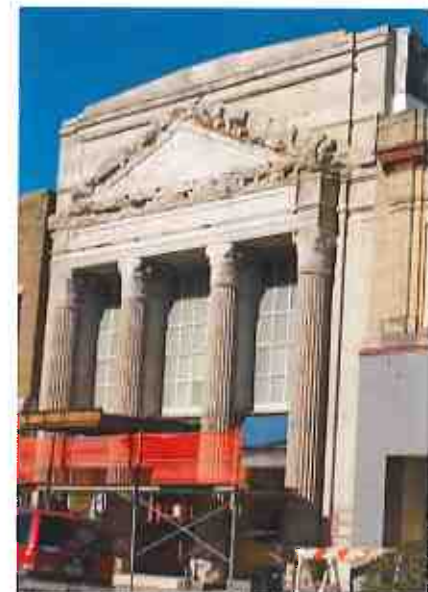
5 West Main Street undergoing renovation
