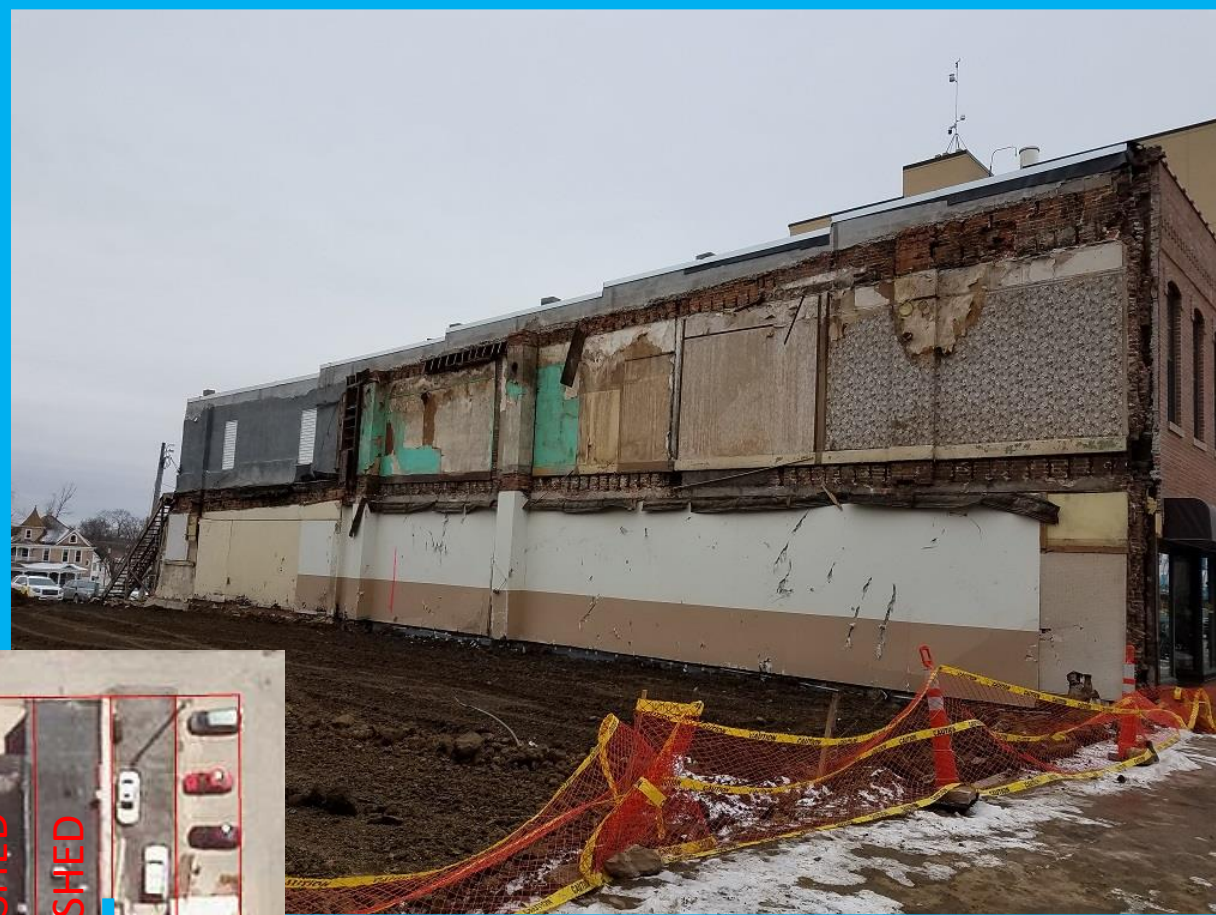
This owner has foundation repair underway and applying for façade upgrade funds to repair the wall and install EFIS.
