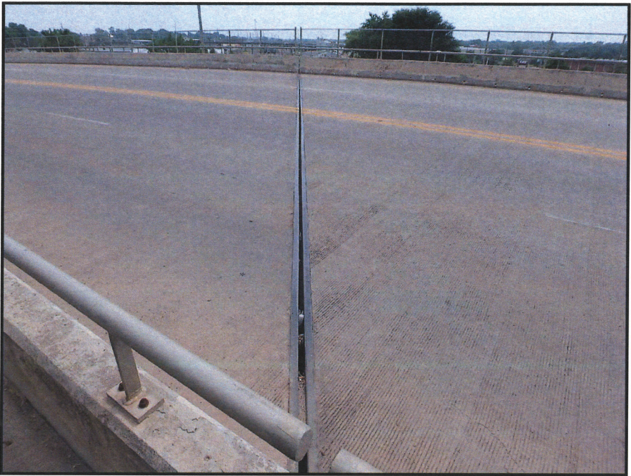
TYPICAL PIER EXPANSION JOINT
