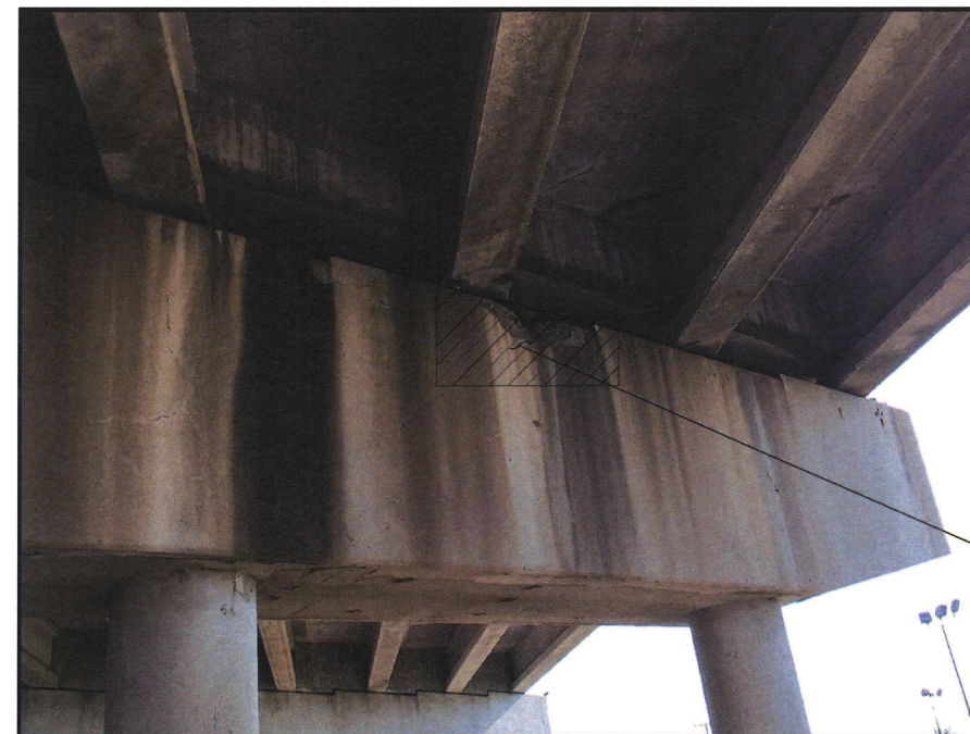
SPALLED SOUTH EXPANSION PIER – EAST END
