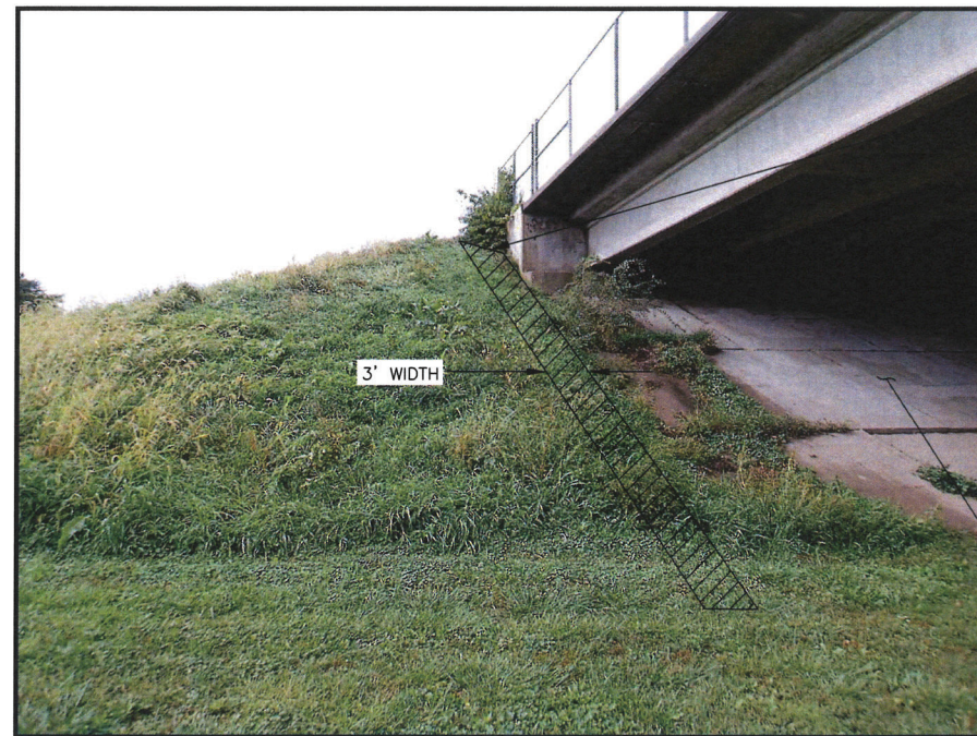
SOUTHEAST EROSION CONTROL REPAIR (TYPICAL @ BOTH SOUTH BRIDGE CORNERS)
