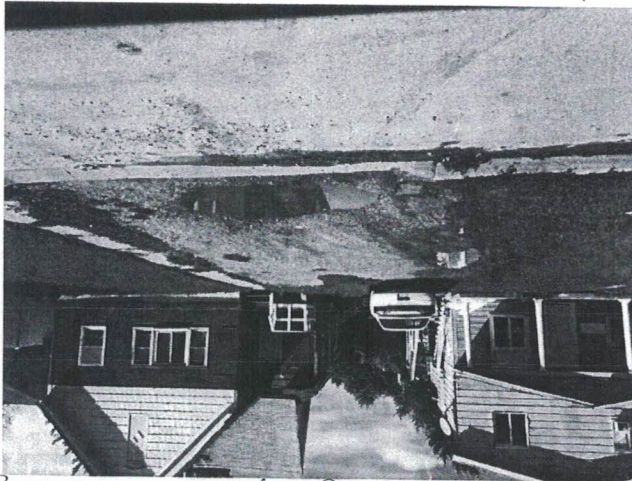
Picture from first inspection and can see that wire does not hold up well – it is bent and distorted as well as coming away with section missing.
