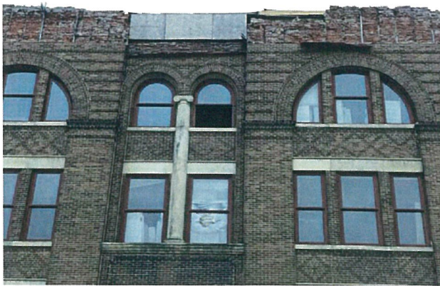
Northern facing façade detail
