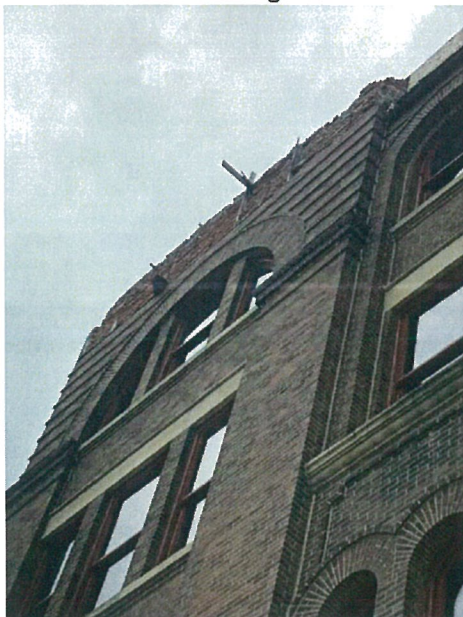
Northern facing façade, top corner detail
