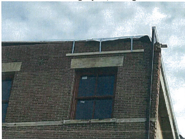
Western facing façade, SW cornice detail
