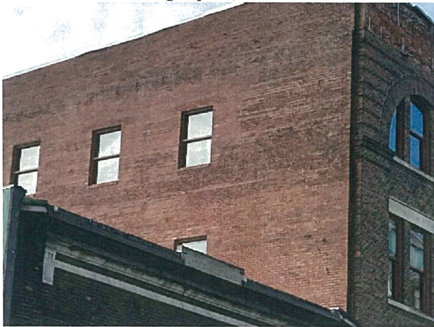
Eastern facing façade, looking west
