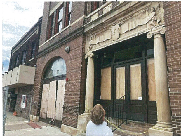
Northern facing façade, Front Entrance
