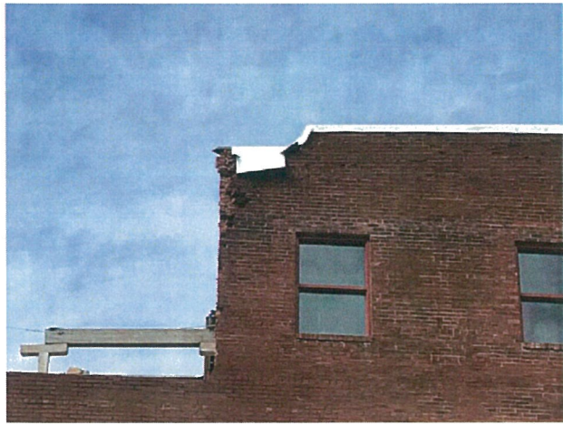
Eastern facing façade, SE cornice detail
