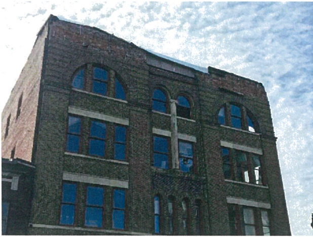
Northern facing façade
