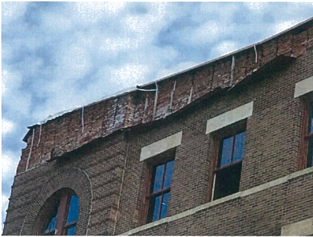
Western facing façade, NW cornice detail
