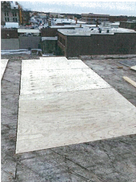
Temporary flooring repair
