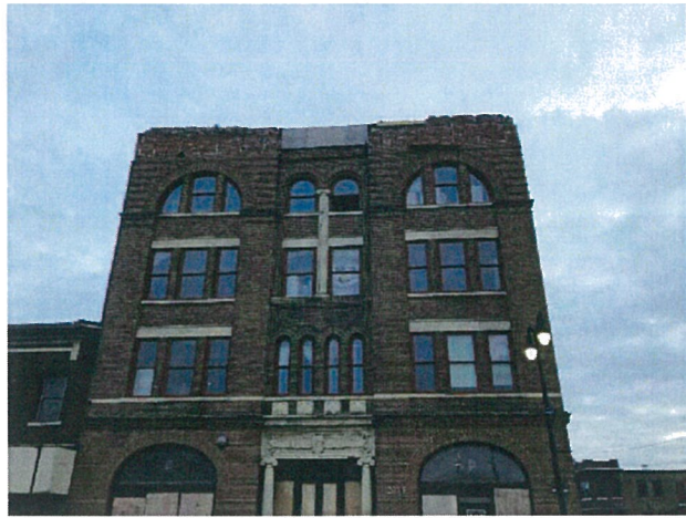
Northern facing façade
