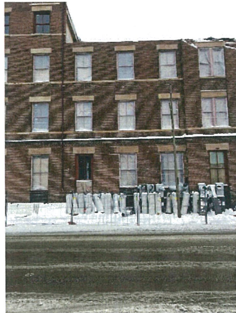
Western facing façade, along E. 2 nd Street
