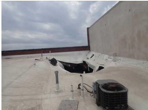
17, 18. Views of collapsed portion and hole in the roof
