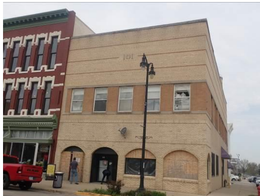
2. View from the southeast
