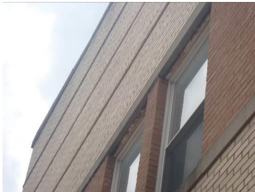
11, 12. Views of rusted lintels
