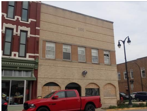
1. View from the southwest
