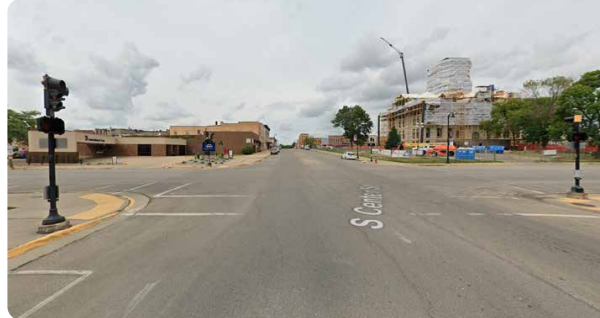
EXISTING CHURCH ST. / CENTER ST. INTERSECTION
