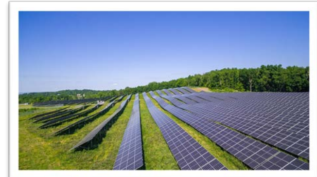
Solar Panels (as primary use)
