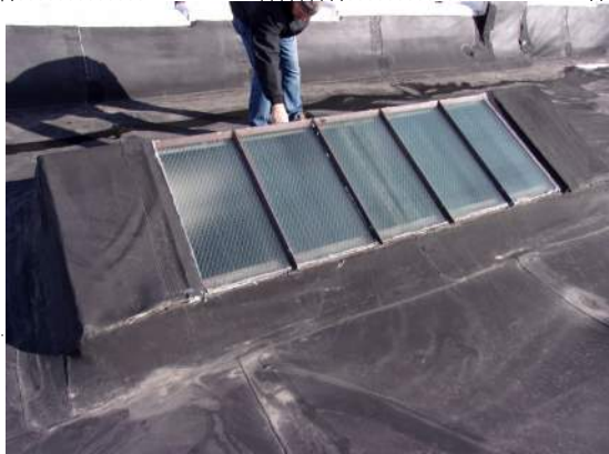
SKYLIGHT AT BUILDING #5
