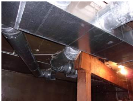
BASEMENT CONDITIONS AT HVAC LOCATIONS.
