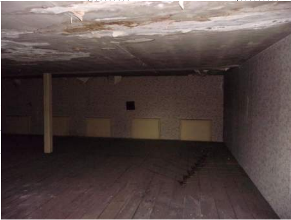
THIRD FLOOR ("MEZZANINE")
