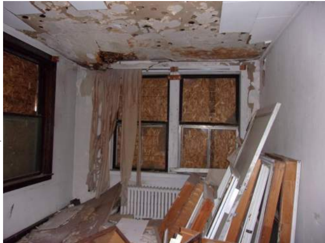
TYPICAL CONDITIONS AT BUILDING #2 AND #3.
