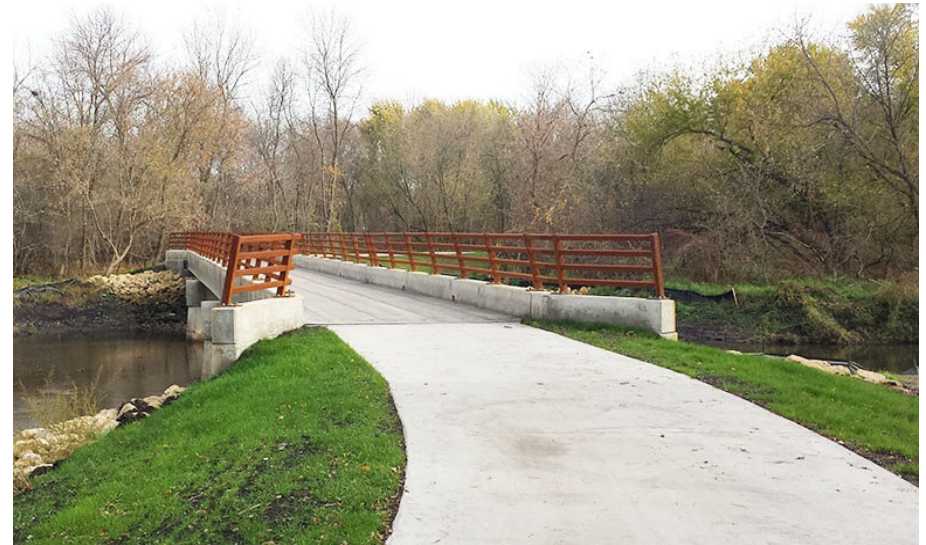
South Troy Park Trail Bridge, Robins, Iowa
