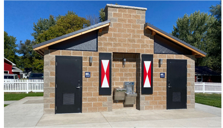
"Dutch"-Inspired Restroom Building, Kiwanis Park, Pella, Iowa
