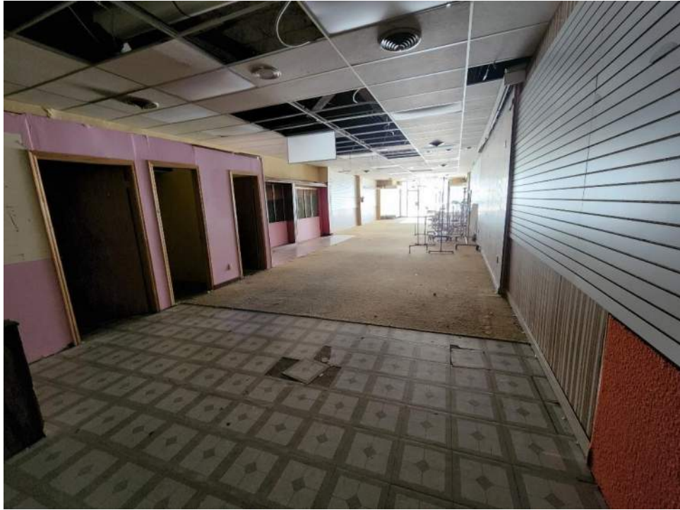
Property Photograph 3 – Rear of main building looking to the front.
