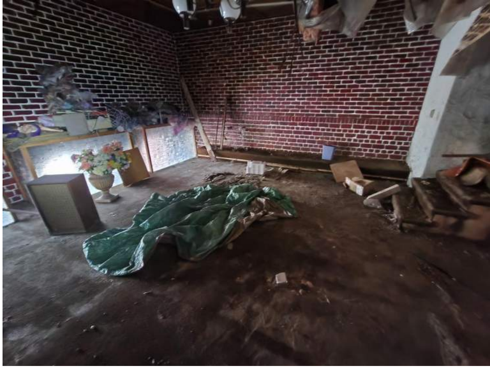
Property Photograph 9 – North room on 2 nd floor.
