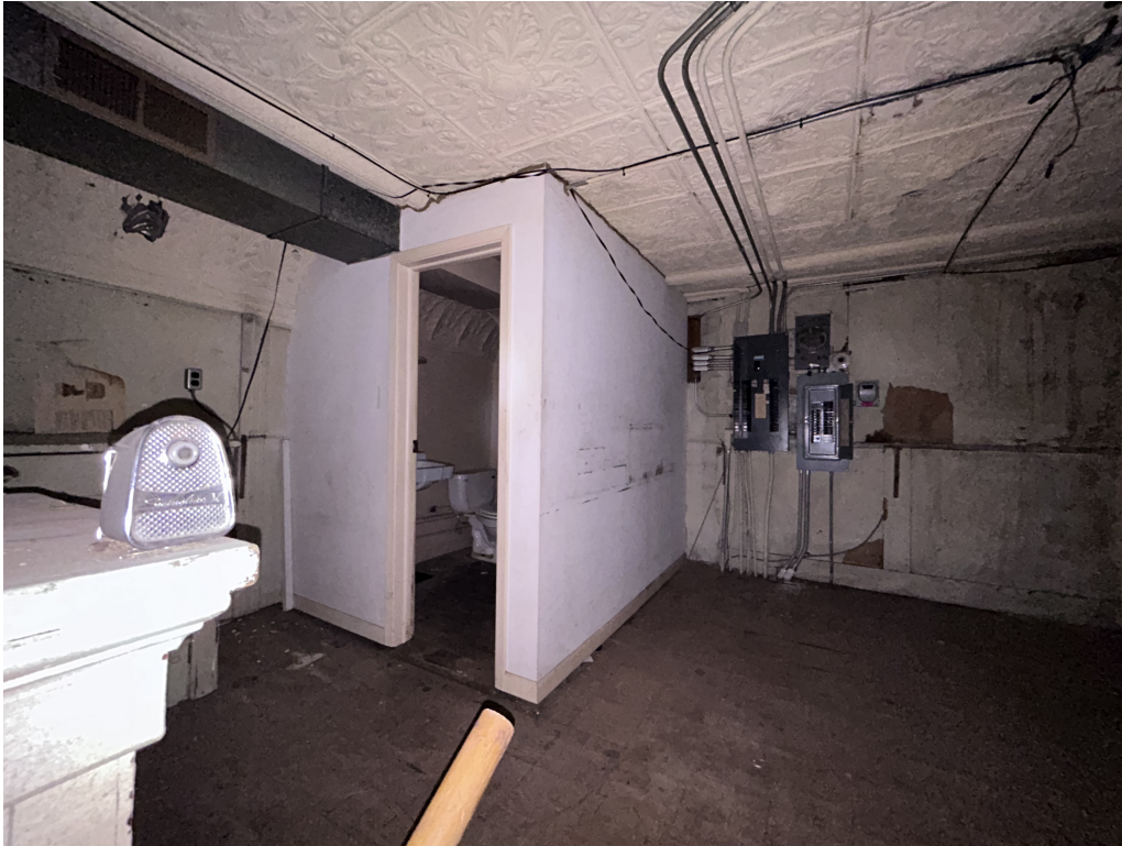
Figure 8 – View of mezzanine bathroom (looking northwest)
