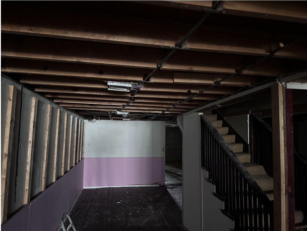
Figure 4 – View of west bay framing looking north
