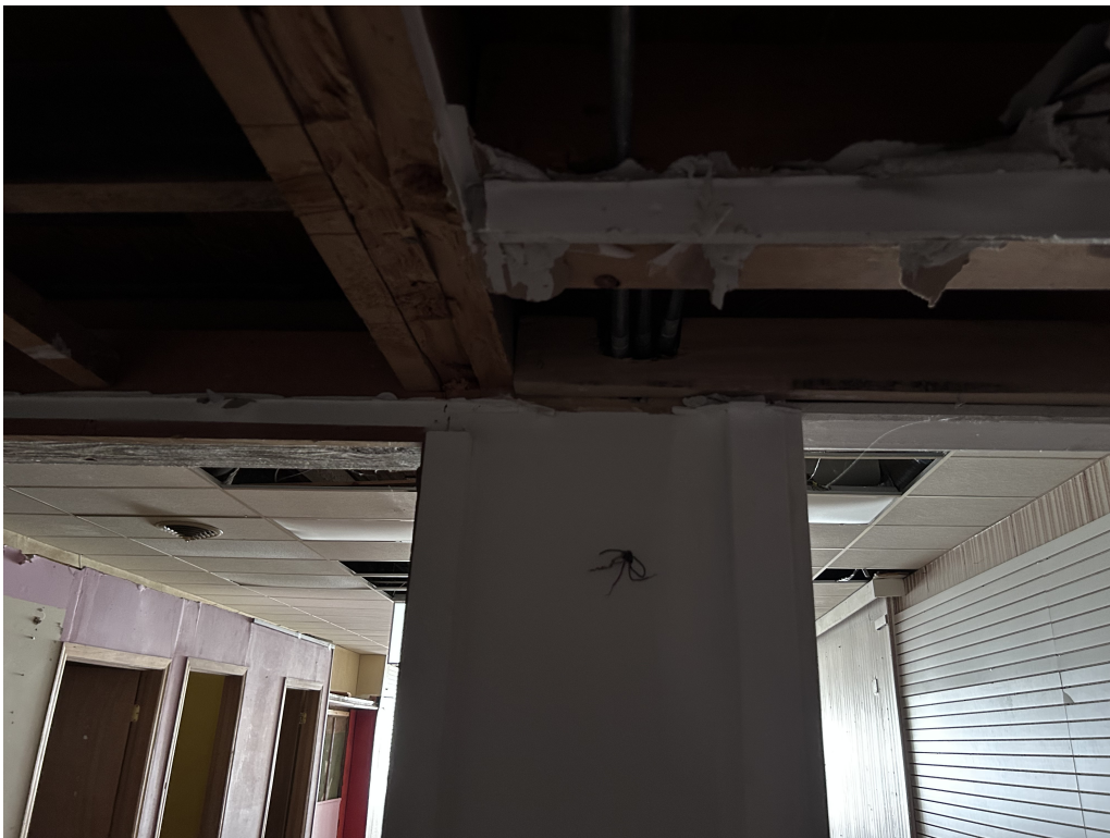
Figure 7 – View of Beam B6 extending over short stud wall. (looking south)
