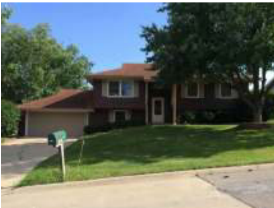
Older single-family detached home (north side)
