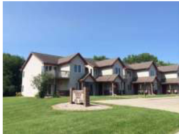
Newer two-story attached homes (south side)
