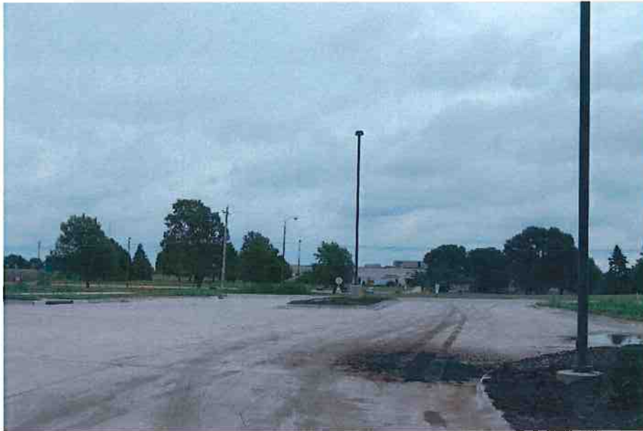
Main entrance/city street looking east from the east property line towards Highway 14.
