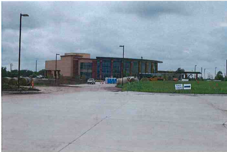
Looking west towards the new building from the west end of the boulevard.
