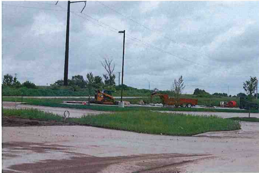
Main parking lot looking north east from Physical Therapy parking lot.
