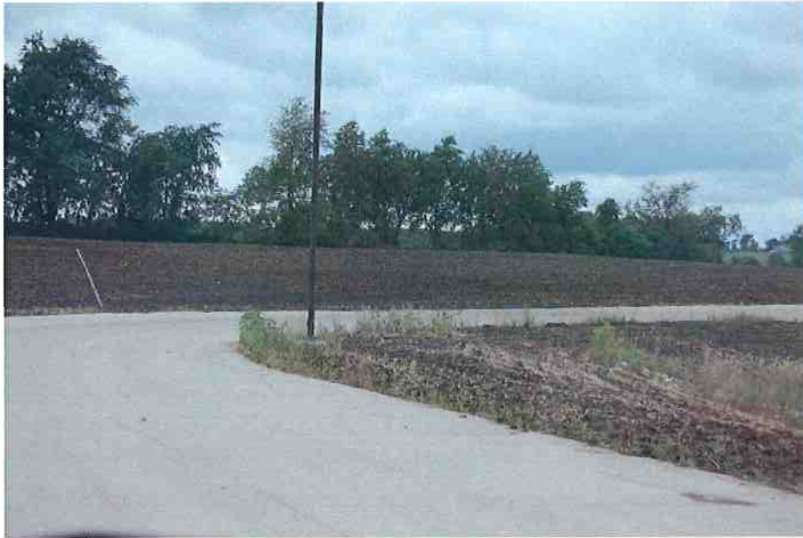
Southern loop road accessing staff parking lot and out-patient pick-up location (looking south west).
