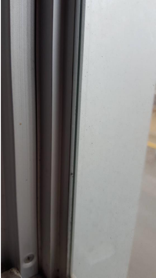
Figure 15: Close-up of existing window frame
