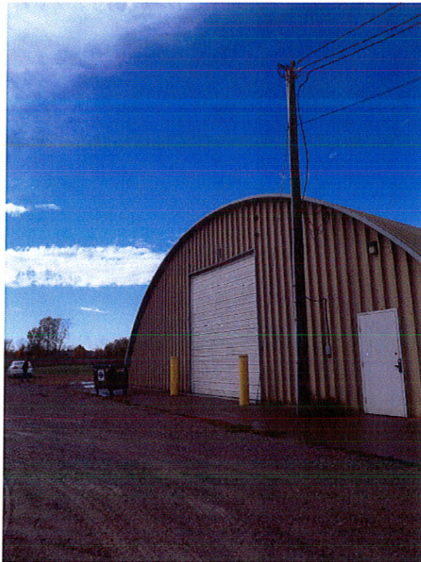
Power Line on Building
