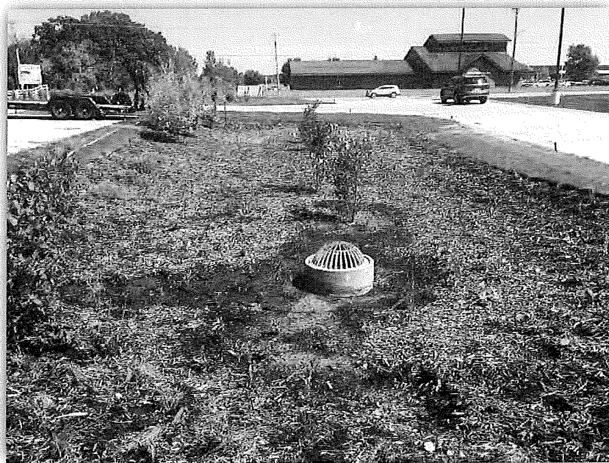
Figure 4.1. Typical Bioretention Cell
