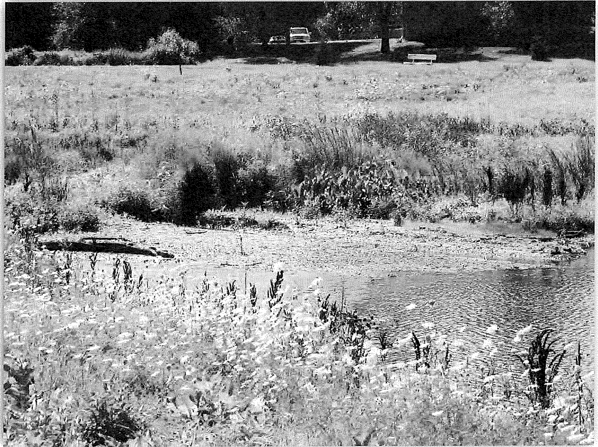
Figure 4.3. Sediment Accumulated in an existing Detention Pond in Timber Creek Park
