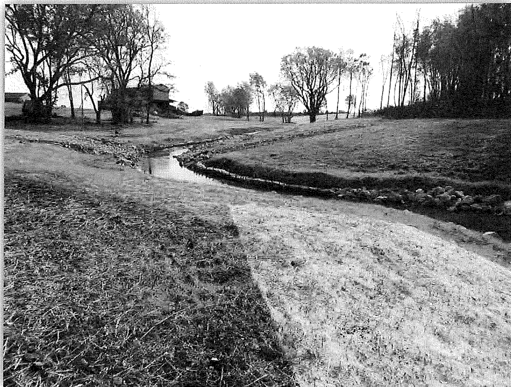
Figure 4.4. Typical Stream Channel Restoration
