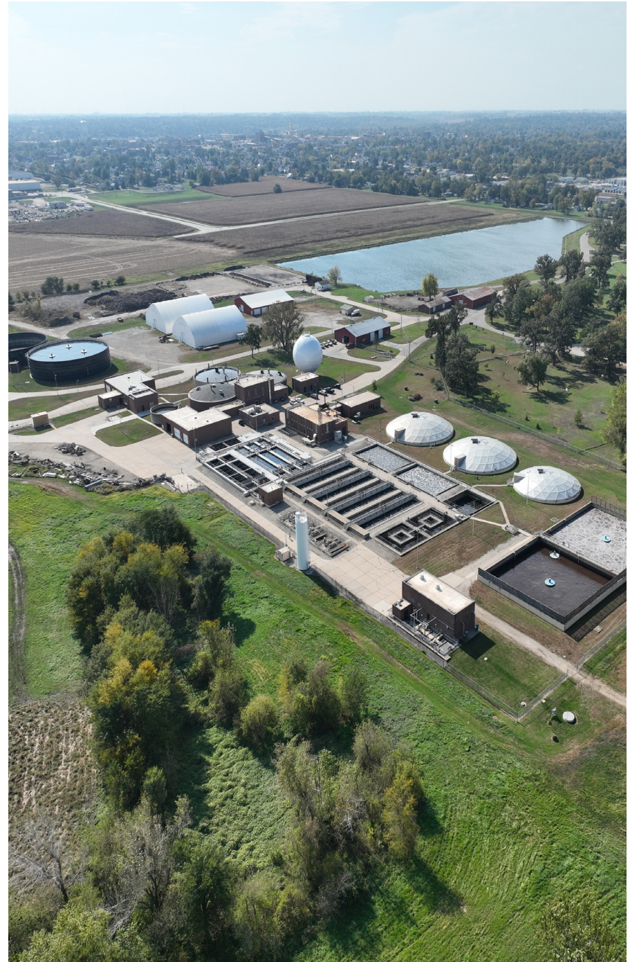
Marshalltown Water Treatment Facility
