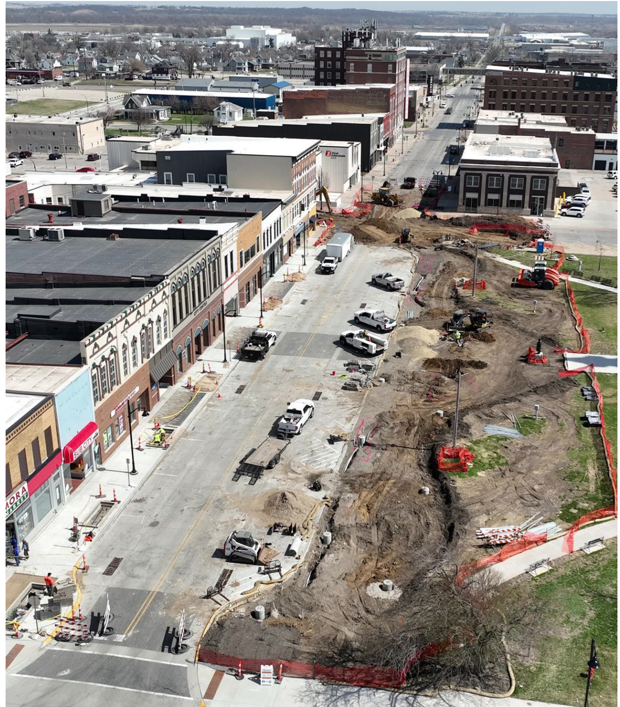
East Main Street Reconstruction, Photo by City of Marshalltown
