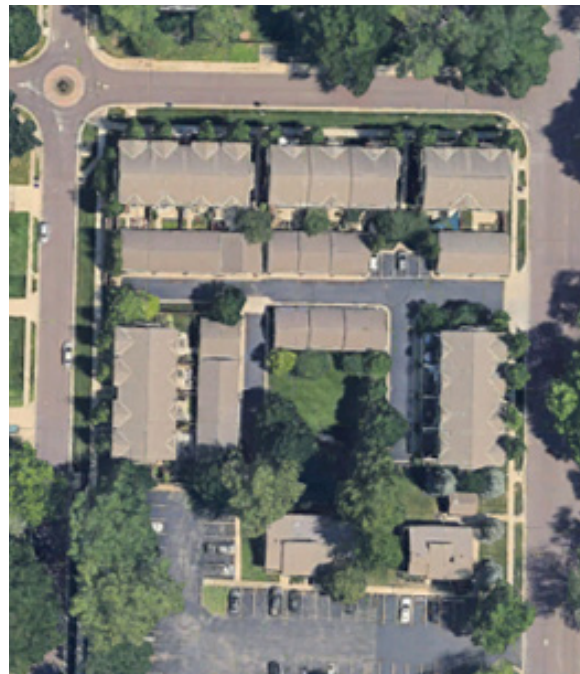
Attached 22 unit Townhome/Duplex Example - Overland Park, KS
