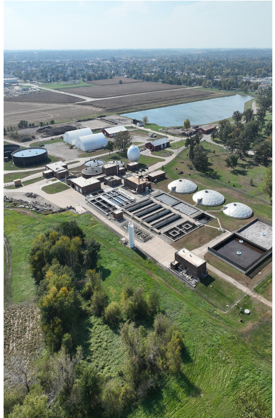
Marshalltown Water Treatment Facility
