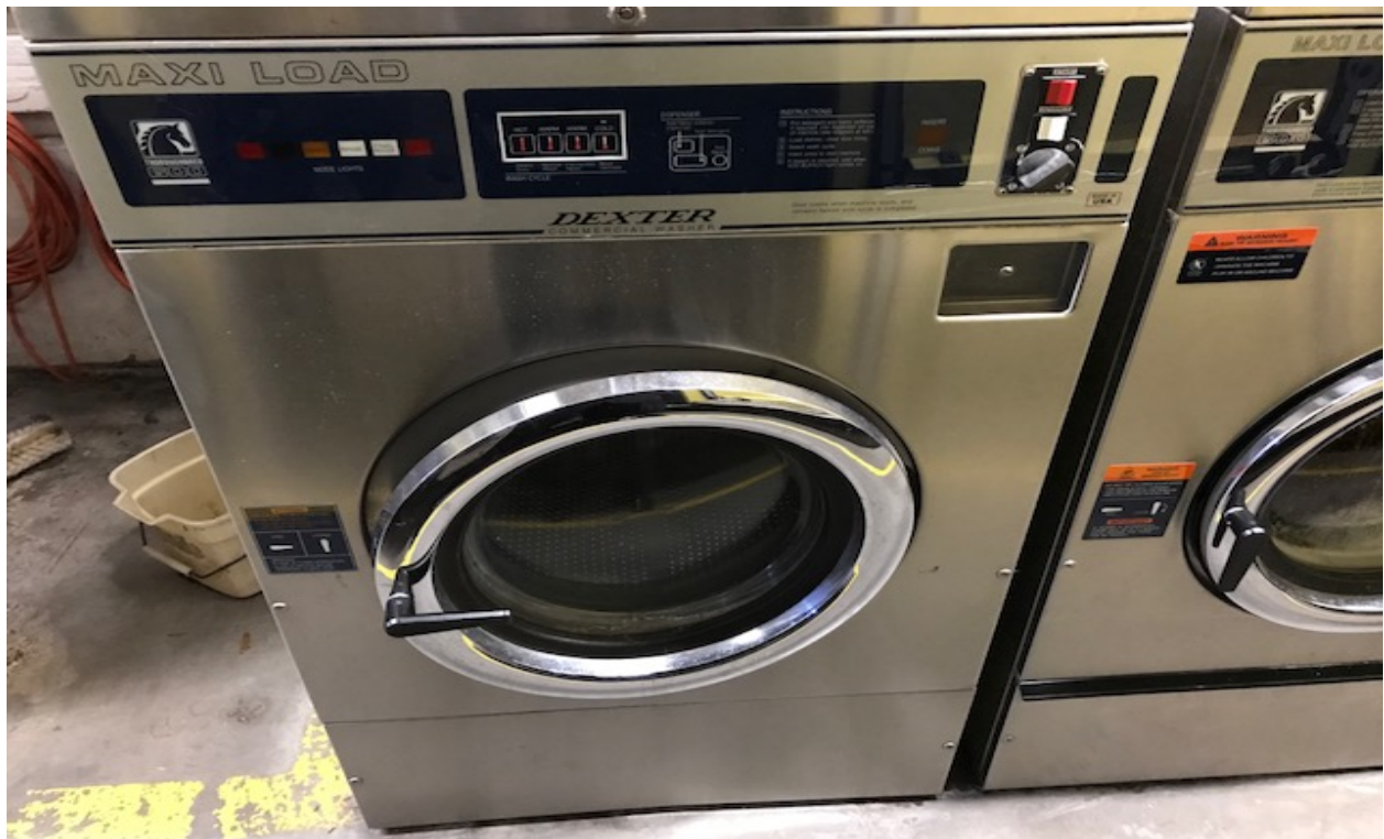
SCBA compressor and fill station and extractor washers being reused.
